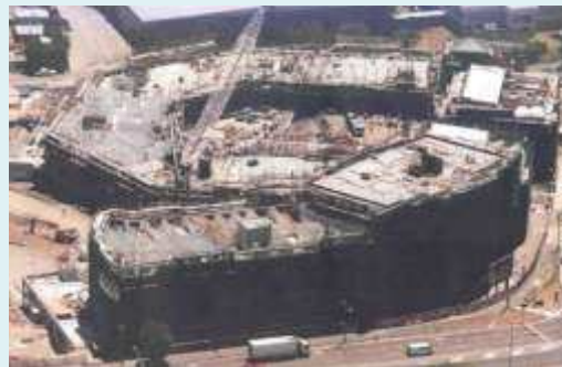
Sydney Park housing complex with 922 apartments. This eight storey building is without RCC columns and beams. The entire structure is built on Gypcrete® /Rapid wall panel.
